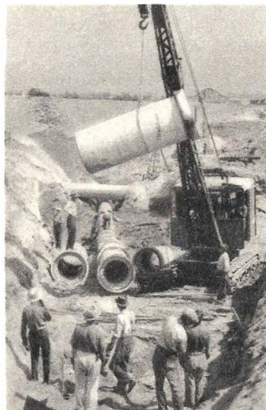
Above—Hinged concrete slab beds and concrete banks are fitted to runaway watercourses so that the water can be carried to specially located spreading grounds where it will gradually be absorbed and stored in subterranean reservoirs. Right—Laying a section of typical aqueduct pipe in place.
