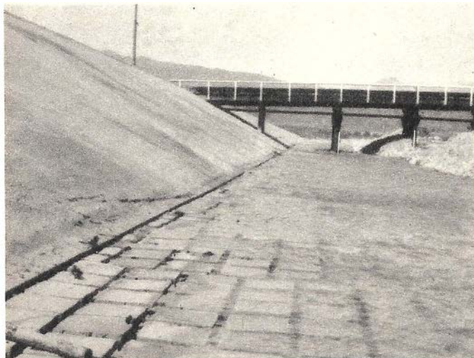
Above—Hinged concrete slab beds and concrete banks are fitted to runaway watercourses so that the water can be carried to specially located spreading grounds where it will gradually be absorbed and stored in subterranean reservoirs. Right—Laying a section of typical aqueduct pipe in place.
