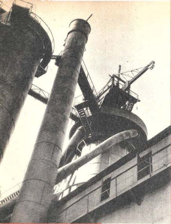
Looking up toward the top of a blast furnace. The first step in the production of steel is the changing of the ore into molten iron. A modern blast furnace produces 600 tons a day.
