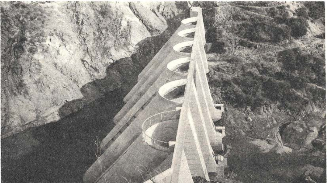
Beautiful curves lend strength to the Big Dalton Dam which impounds drinking water for the Los Angeles County area.
