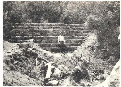
Left—This large city reservoir is small when compared to the huge underground storage basins created by engineers. Above—A rock, wire and brush check dam that serves to slow the onrush of water down a mountain side, allowing it time to soak into the ground.
