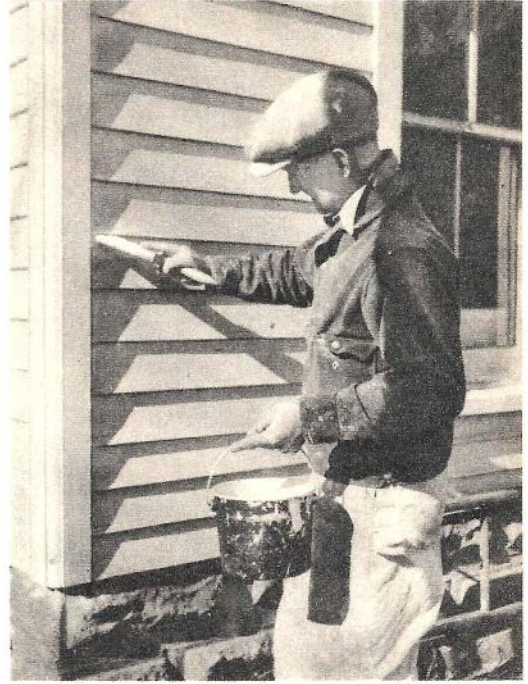
The proper method of applying paint is as follows: Dip the end of the brush into the paint; slap it lightly against the side of the pail, and give the brush a half turn before applying it to the surface. This prevents paint from dripping from the brush. Work it out with the grain, and then across the grain. Finish with light strokes with the grain.
