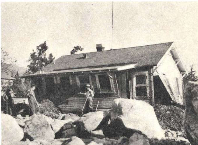
Above—This home was wrecked as a result of a cloudburst near Montrose, Calif., before proper flood control methods to divert rain waters into the ground were adopted. Left—An engineer using a device that gauges a river's rate of flow.
